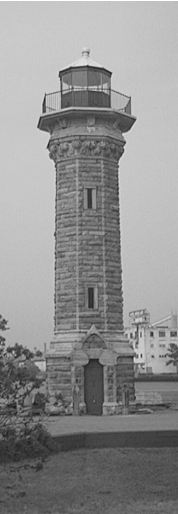
Lighthouse Restored Major parts of the restoration of the Island’s landmark lighthouse have been completed. The cleaned stone appears lighter. Remaining to be done: Slate walkway around the structure’s base, plus interior and exterior lighting. The project was funded by Friends of Roosevelt Island Landmarks, Inc.
