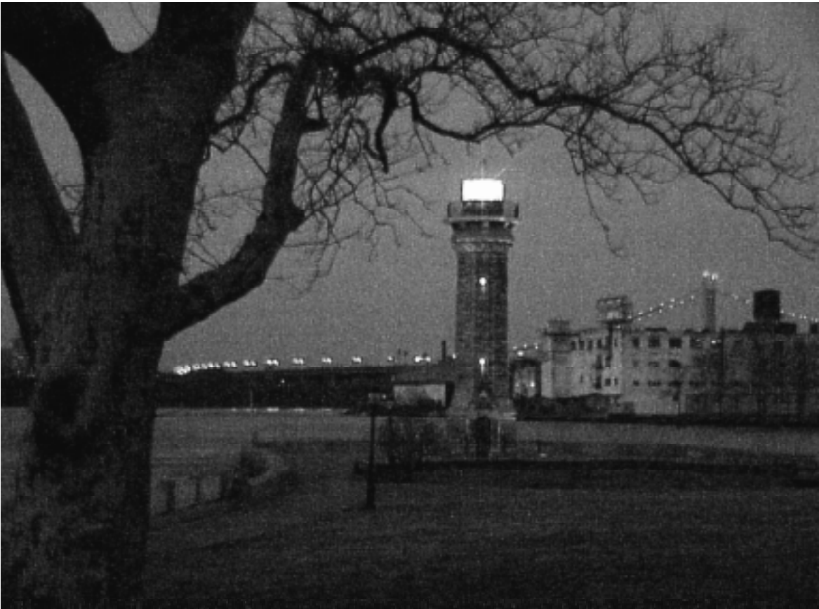
Roosevelt Island's northernmost landmark is once again a lighthouse in every sense of the word. Newly restored and reilluminated, it was the centerpiece jewel in the necklace of the Triboro Bridge Wednesday night at dusk.
