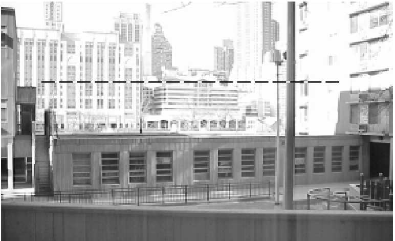
View from the Island House courtyard shows the one-floor mini-school that would become a two-story structure under the conversion planned by Diane Wilson of Corporate Realty Partners. The line approximates the top of the proposed second floor.
