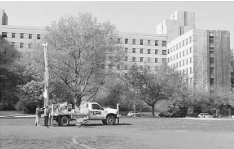
Website NYC10044 www.nyc10044.com This rig drilled to bedrock last week on the soccer/baseball field just north of the Nurses Residence in preparation for Southtown construction. The 13 holes found solid rock at depths ranging from one foot to as deep as 52 feet, and, according to the men operating the equipment, discovered an area with "lots of fill," possibly where native rock was quarried in the 19th Century to build a number of Island buildings, only a few of which remain today. The workers also drilled for a core sample of the bedrock for analysis.
