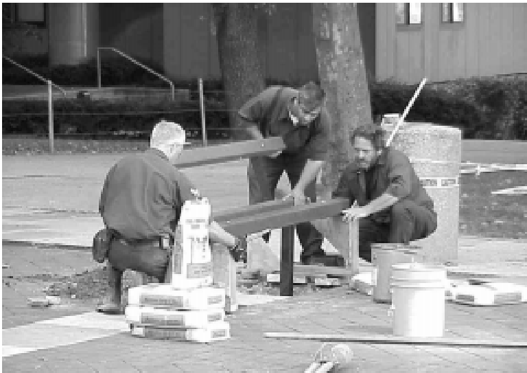
New Benches were being installed by a RIOC crew Thursday afternoon at the west end of Good Shepherd Plaza.
