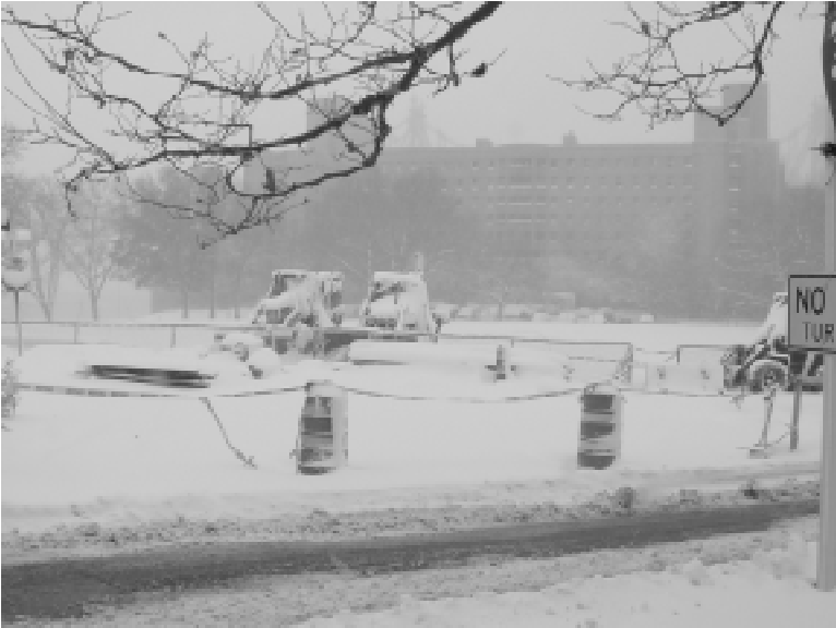
Snow covered construction equipment last week at the Southtown site where the west roadway is being widened. In the background is the long-vacant CNR, or Central Nurses Residence, due to start coming down within a few weeks.
