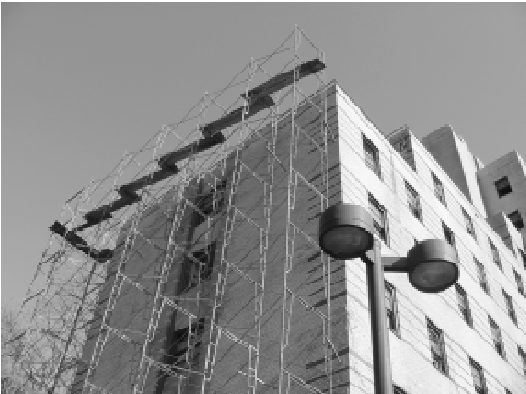
Demolition Starting Scaffolding rose last week at the abandoned Nurses Residence, which is due to come down soon as part of the Southtown construction program. A fence is also being erected around the site, and the west service road is being widened for two-way traffic. The east road is to be eliminated.
