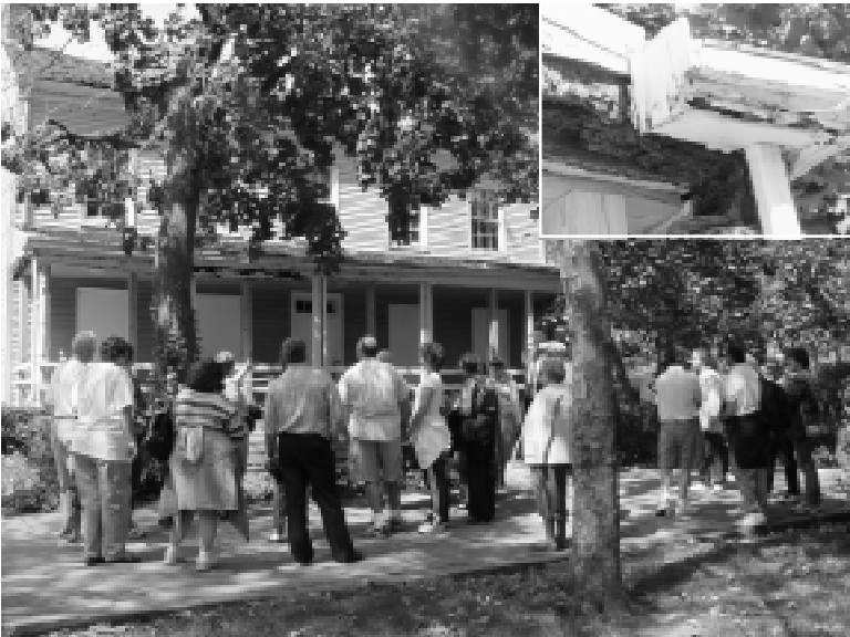
A Gathering of Blackwells Some three dozen Blackwell family descendants gathered on the Island last Sunday. Historical Society President Judith Berdy gave them a tour that included the deterioration (inset) of their ancestral home, which several of the visitors were seeing for the first time. Later, they plotted strategy for returning the house to fully-restored condition. On Thursday, the RIOC Board will approve another attempt to get State historic preservation funds for the house; RIOC's first application was turned down.
