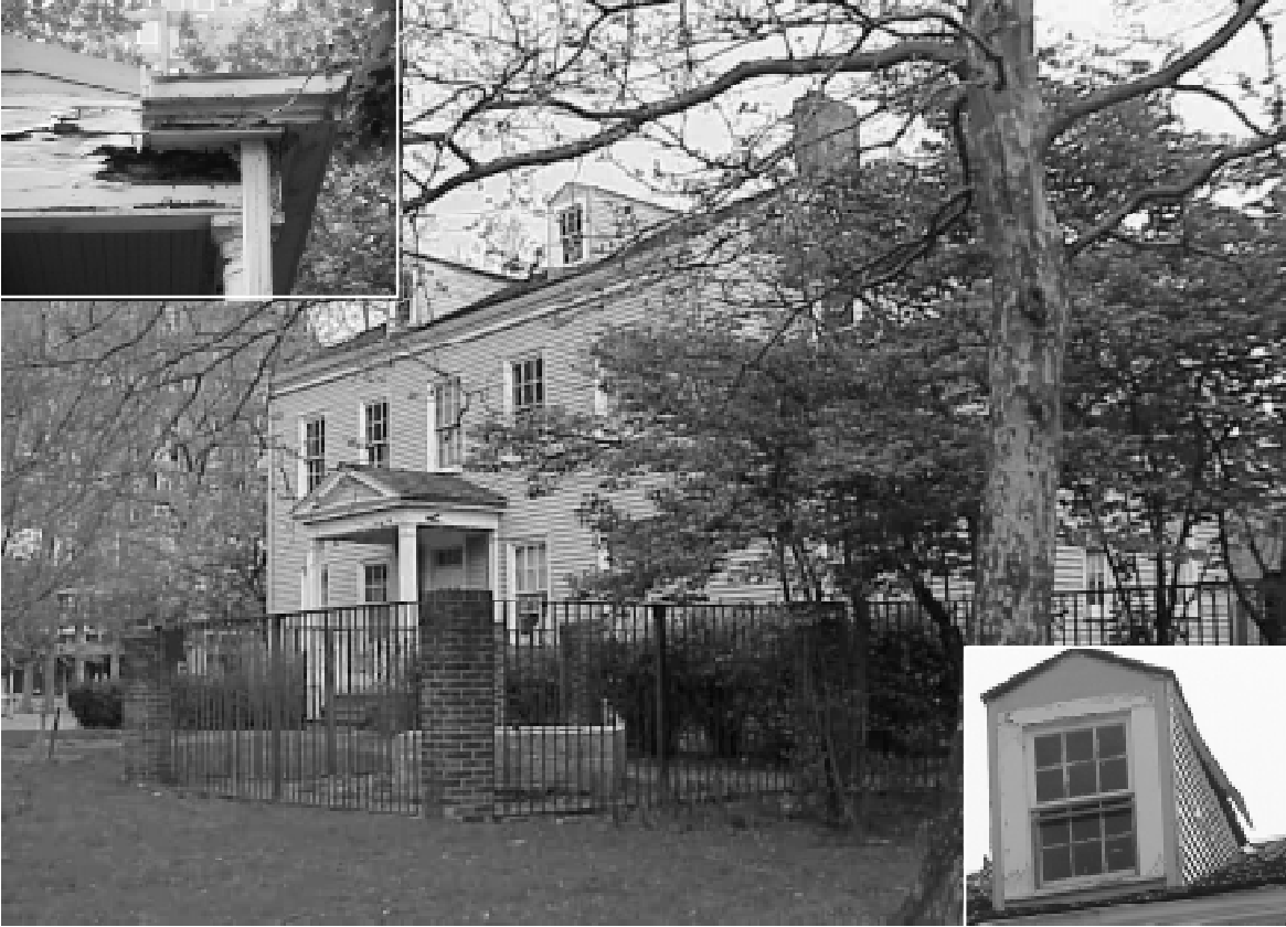
Historic Blackwell House, with inset photos of serious deterioration on RIOC's watch
