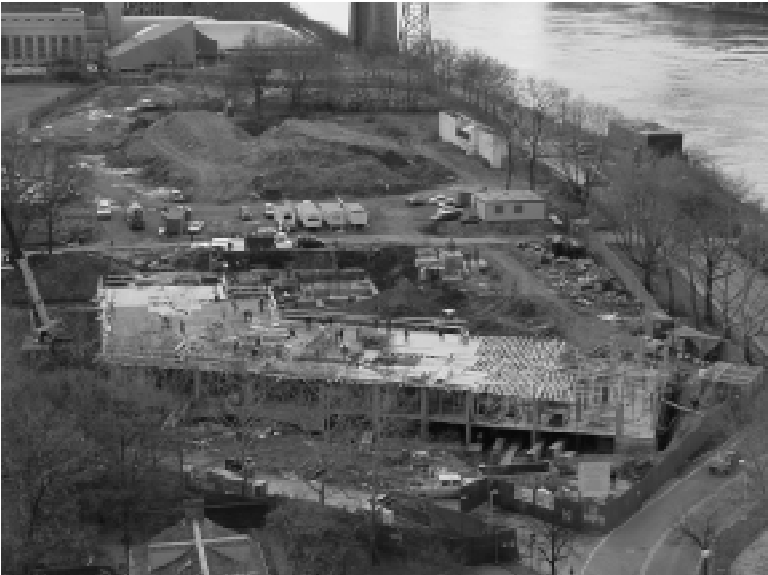
Southtown’s first building finally rose into view above the fences in the past week. Photo taken from Eastwood shows the structure’s footprint and, immediately behind it, the beginning of infrastructure construction for the second building. More photos, in color, on Website NYC10044 at www.nyc10044.com .
