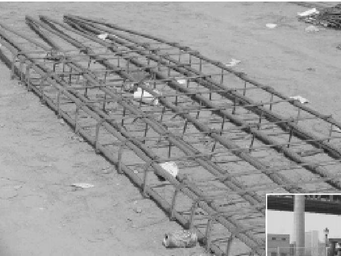
Reinforcement bar – rebar – is built to shape on the Southtown site. Rebar crews like the one at upper left form it, then wire it together. The shapes are then transported to the building, where they are embedded in concrete to form columns and floors.
