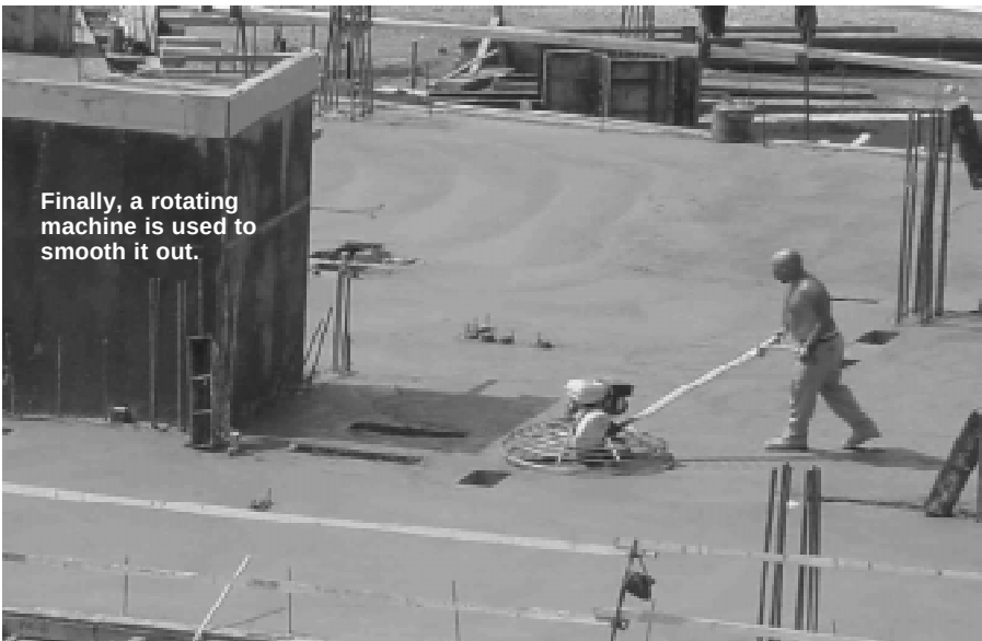
The sequence of photos at the right shows the completion of a floor.
