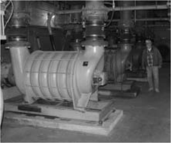
Many centrifugal fans (left) inside each of six exhausters (above) create the suction that creates a 60 mph wind to pull residential refuse through underground pipes to the AVAC building.
