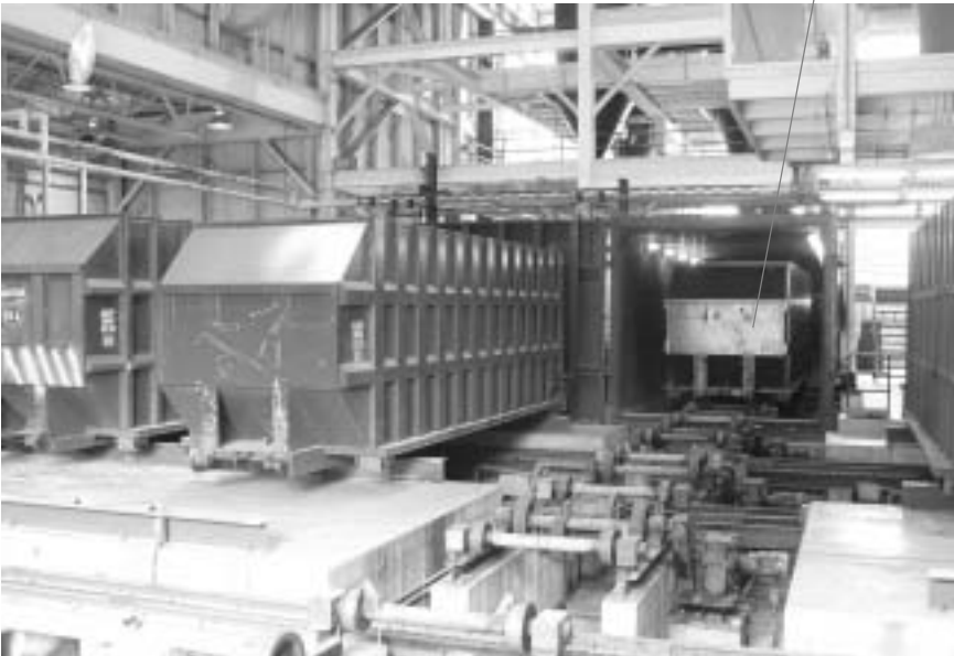
...that sits atop a collection chamber dropping waste into a storage container.
