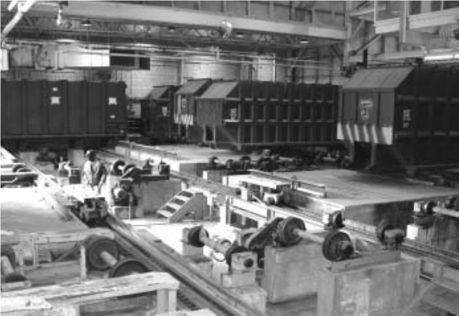
Containers are shuffled into position and onto trucks on a system of rollers. Doors to trucks pulling up outside are located out of frame to the left in this photo.
