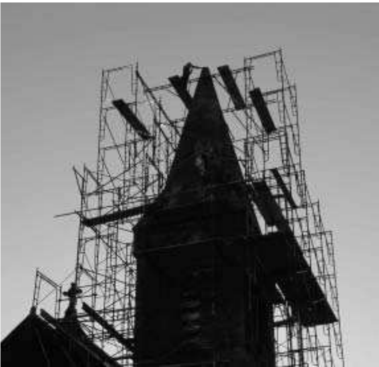
The steeple of the Chapel of the Good Shepherd gradually disappeared this week, hidden behind scaffolding, then safety net. A worker seemed to be touching the peak as he surrounded the structure with a platform to be used by restoration workers.
