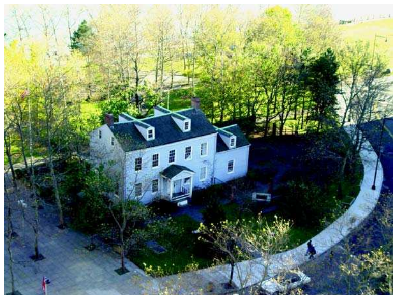
Blackwell House falls under the long winter shadow of 475 Main Street, the northernmost building in Southtown. The oldest structure on the Island, the farmhouse is long overdue for repairs, its bowed roof evident in this photograph. The Historical Society is working with RIOC to move the process forward.
