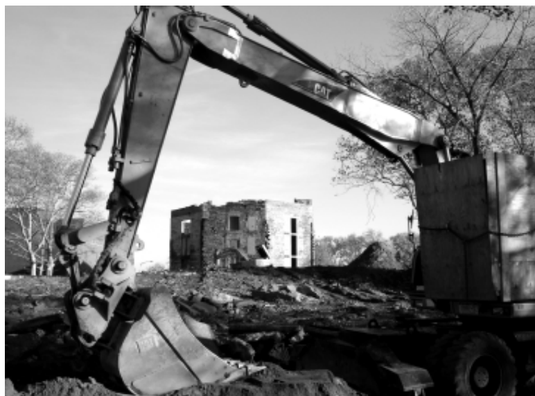
The Octagon Tower was framed by construction equipment Tuesday afternoon as site clearing progressed. More photos, page 6, and in color on Website NYC10044 at nyc10044.com .
