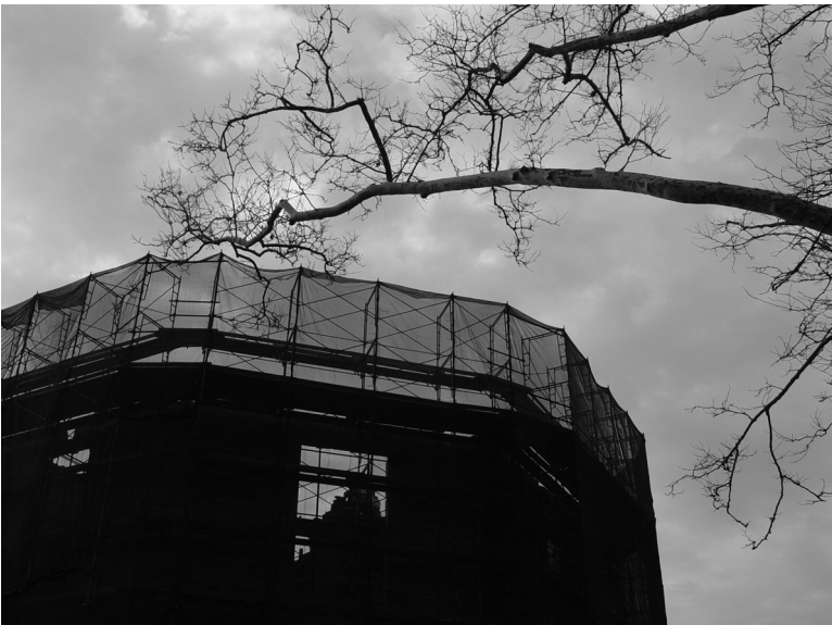
The Octagon is now fully wrapped, as work continues on restoration.
