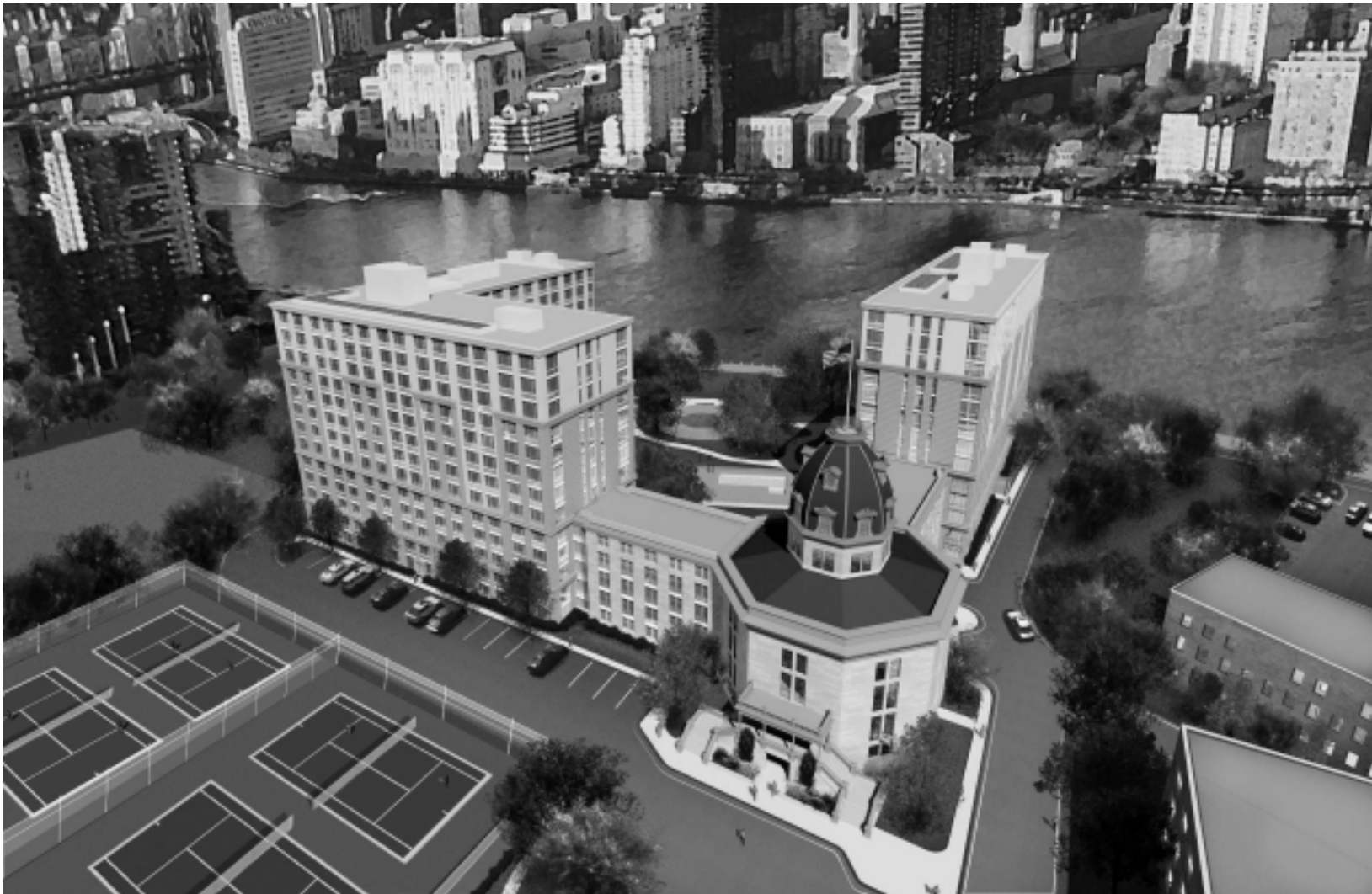
Becker and Becker Associates, architects of the Octagon Apartments project, released this aerial rendering of the project last week. Bruce Becker said construction is going smoothly, "and if the cold weather lets up, the Octagon restoration work will move even faster." Completion date is projected for the end of 2006, but "the tennis courts are being rebuilt by us and should be back in use by this summer, assuming construction continues without any interruption." He said plans are for the Red Bus to stop in front of the building, adjacent to the courts.
