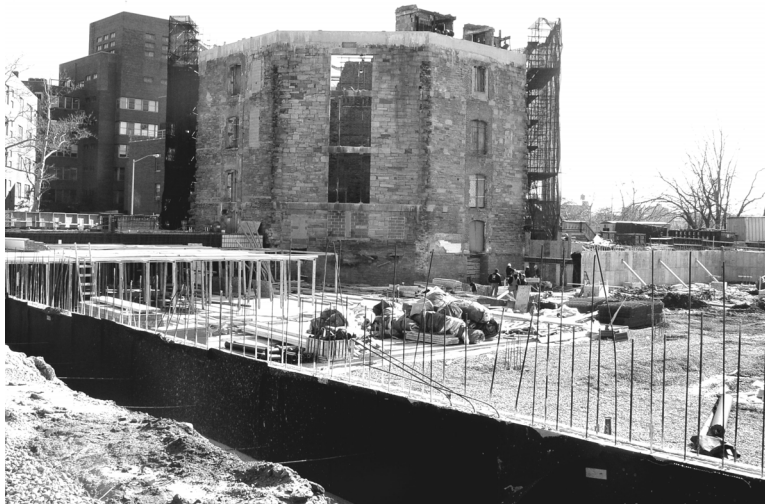
Excavation for the Octagon Apartments project now appears complete. The foreground area will be part of an underground garage. The top of the Octagon tower shows a new, lighter-colored finish where restoration work has been done. To the left, Coler Hospital rises behind the tower.
