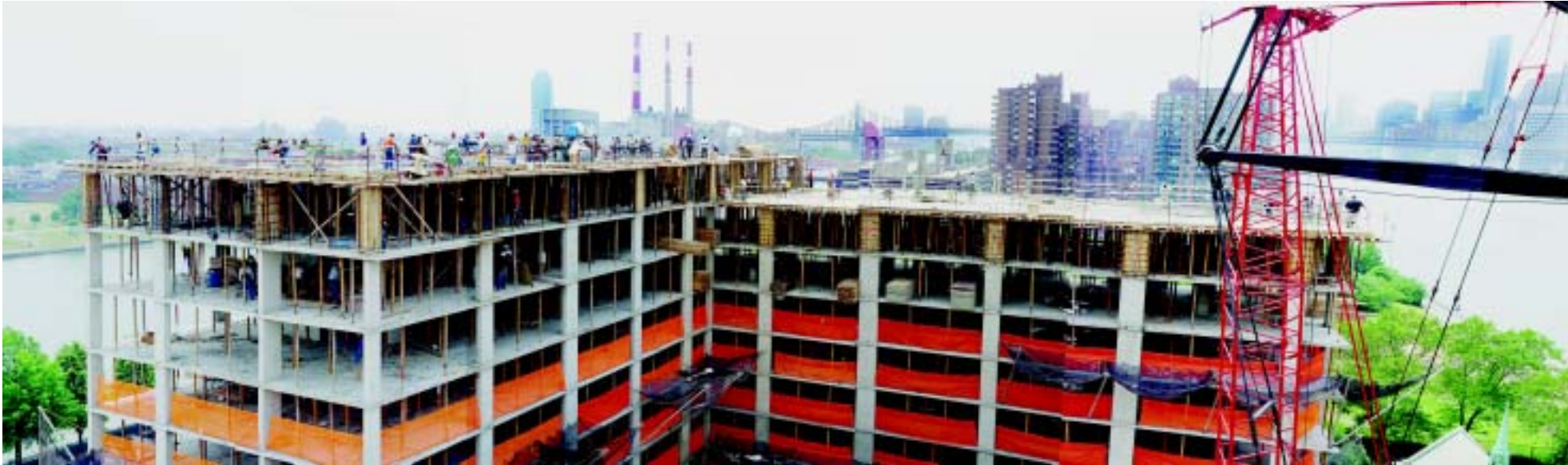
From the Octagon Apartments' north tower, which was finished first, a swarm of workers can be seen finishing the east tower. There are panoramas of the view in this issue's center spread. The project employed over 1,000 workers. The project will be owned by The Multi-Employer Property Trust (MEPT), a real-estate fund that pools over 250 pension funds to invest in such properties. Looking south, in the background are the Citicorp Tower in Queens, Keyspan's Ravenswood power plant, the Roosevelt Island Bridge and Queensboro Bridge, and the Manhattan Park buildings. To be added to the list for the 100 affordable apartments or the 400 market-rate apartments, call 888-292-4990 . Panorama assembled by Paul Katz
