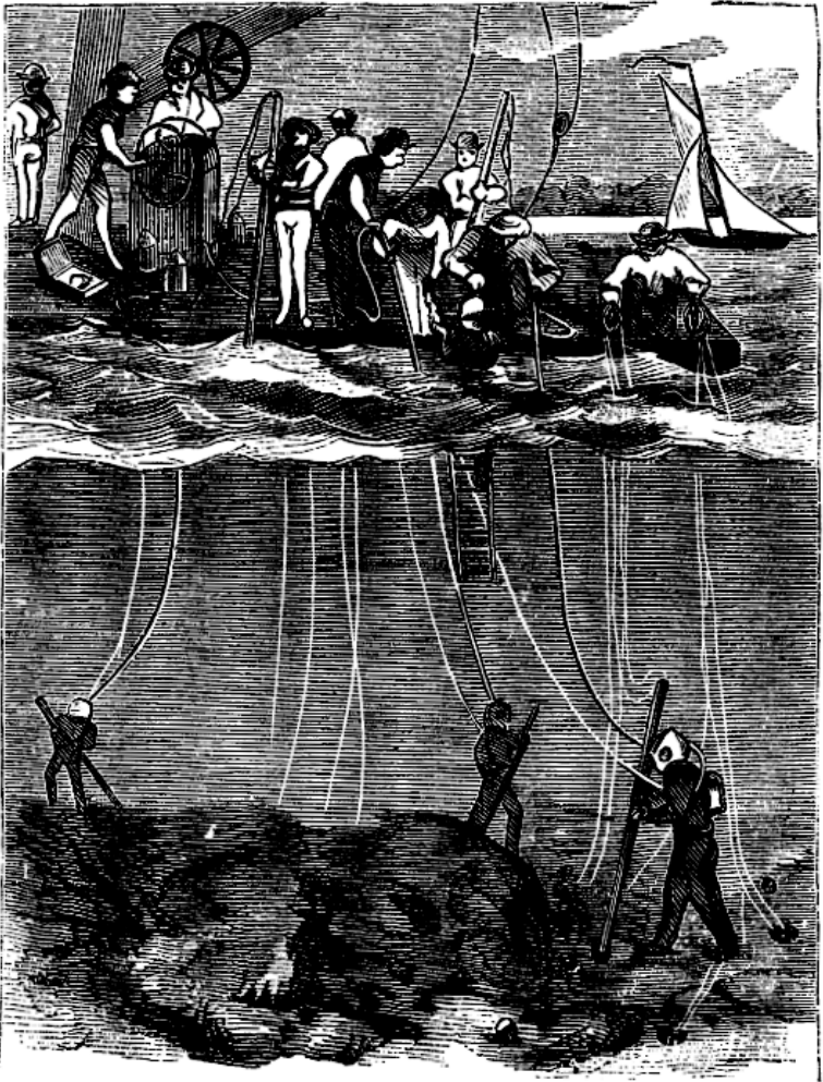
Divers drilling rock
