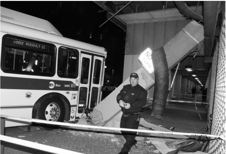
Pulling up to discharge passengers, a Q102 bus nudged a non-support pillar into the Eastwood walkway last week. Nobody was hurt.
