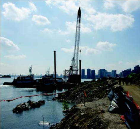
Below, barges bearing the blocks of granite, and the crane that transferred them (as in the photo at right) to the construction site.
