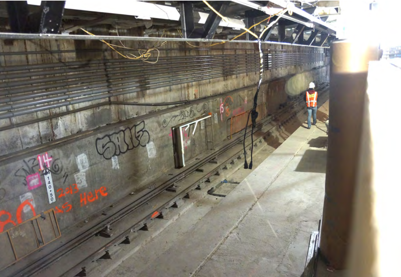
This is what you’d see if those blue-board construction barriers were down at 63rd and Lex. It doesn’t look like much now, but in a couple of years, the tracks will carry the Q train, and passengers will be able to transfer cross-platform between the F and the Q.
