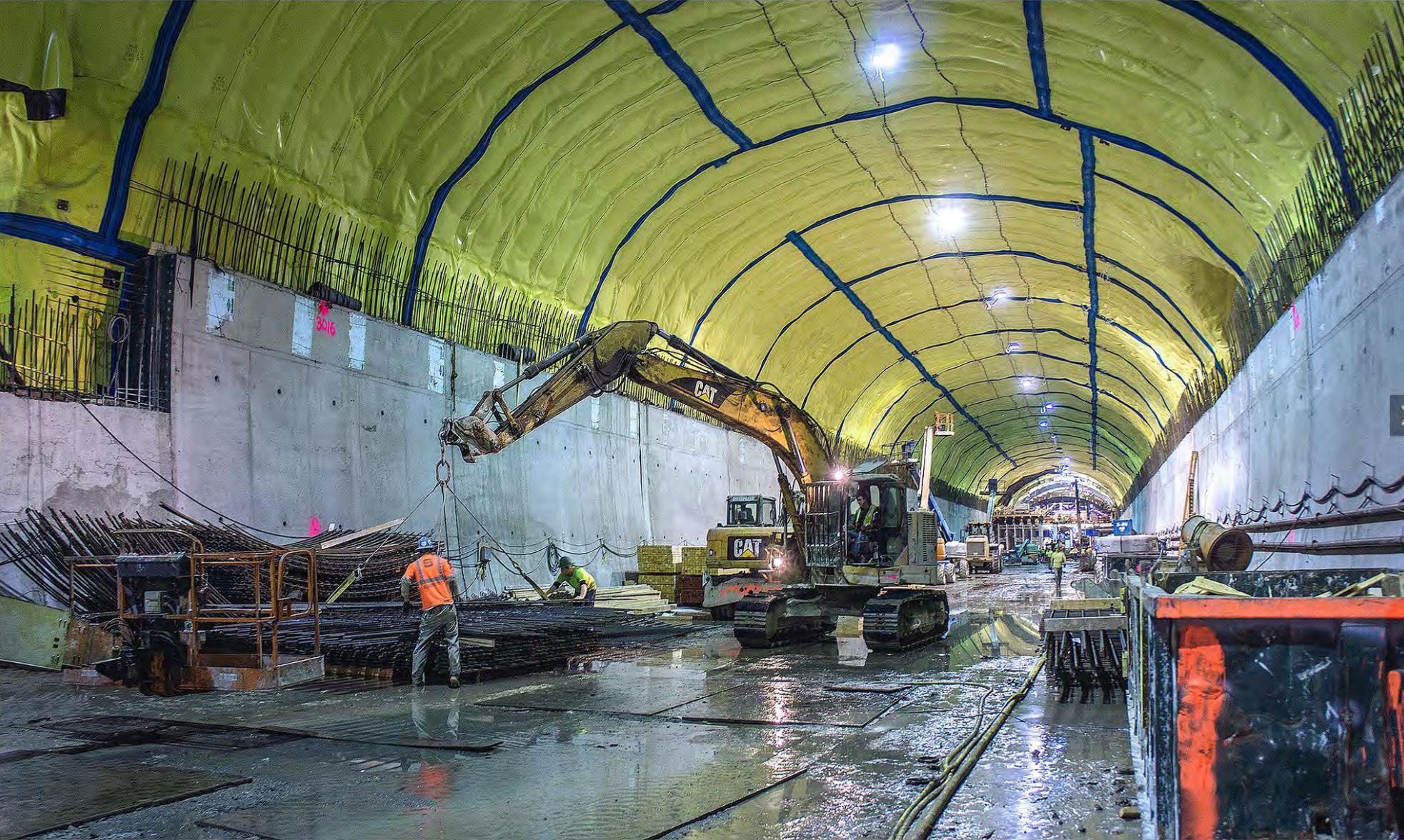
Arc of cavity top gives a sense of the size of the T/Q line’s 72nd Street Station in this MTA photograph. More are exhibited on its flickr site, accessible via tinyurl.com/2ndAvMTA .
