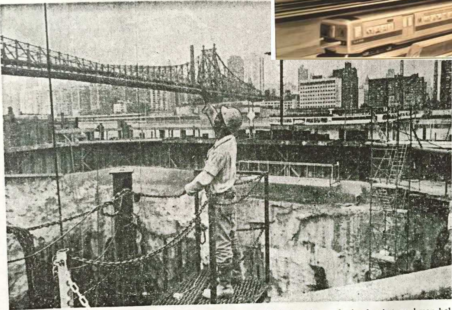
From platform extending over 110-foot-deep hole on Welfare Island, sandhog William W. Jackson Sr. of Brooklyn directs operator of crane, unseen at left,
